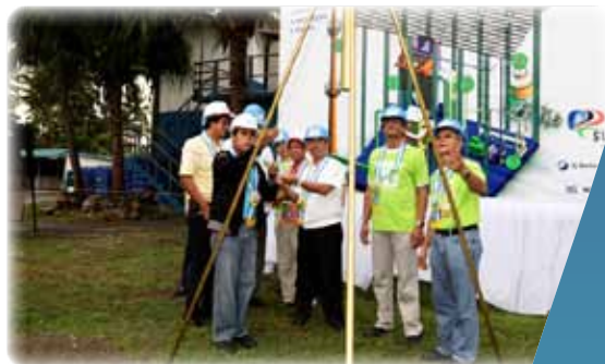
Breaking ground on a biomass cogeneration plant in La Union Province, the Philippines (May 28, 2010)
